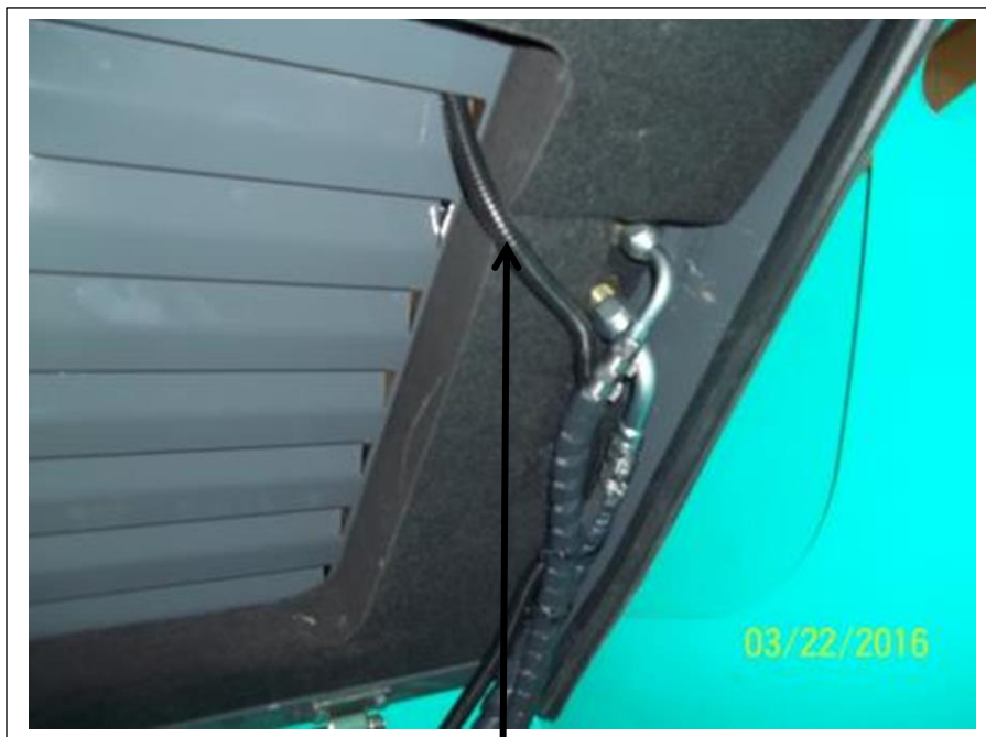
#6 straight fitting from bulkhead
